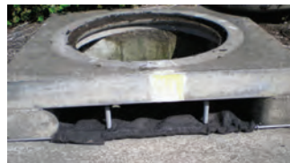
Outside View Curb Inlet Unit
